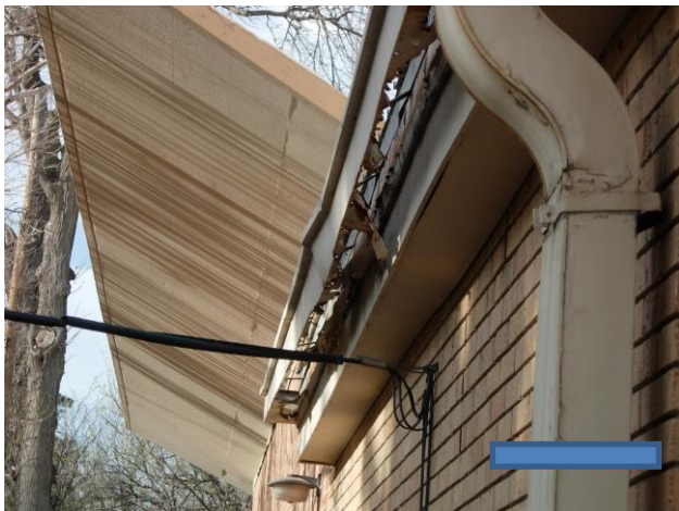
West guttering of church
